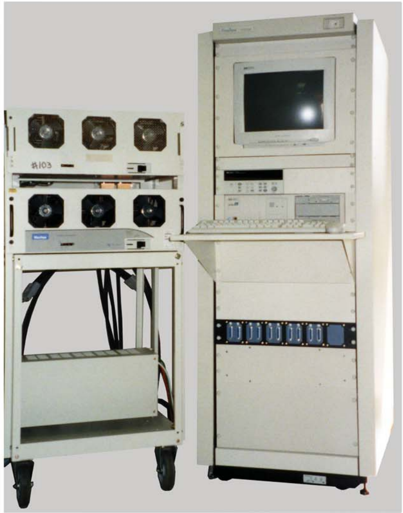
Burn-In Monitoring System and Cart with 2 UUTs
